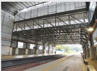
Pembinaan Platform 1 & 2 Construction of Platform 1 & 2
