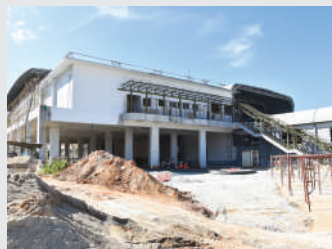
Pembinaan bangunan stesen Construction of station building
