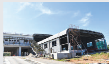
Pemasangan Portal Frame Installation of Portal Frame
