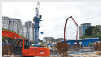
Pembinaan raft foundation Construction of raft foundation
